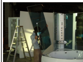
17. Installer glass venstre side
